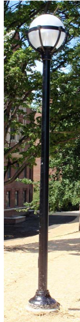
typical pedestrian scale light pole
